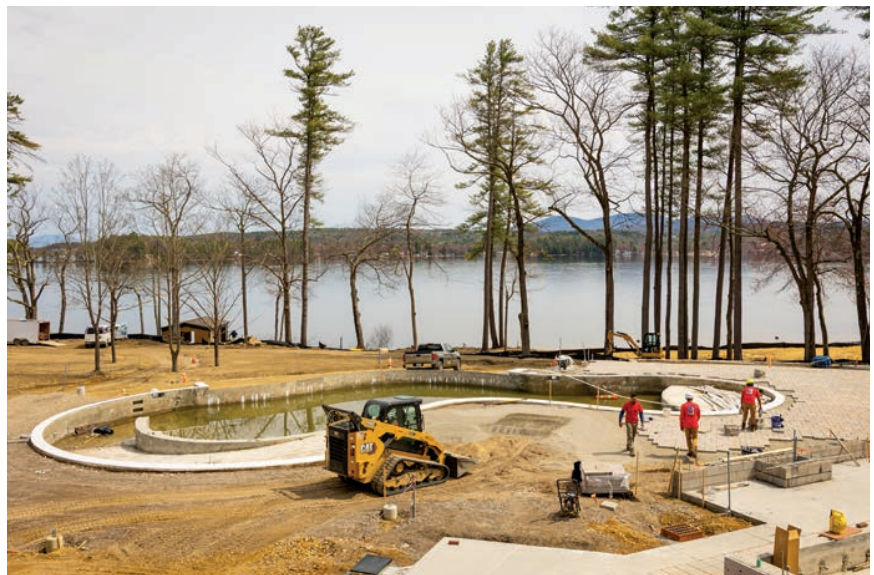
The pool area overlooking the lake, under construction in April, includes a “bourbon room” in a boathouse by the shore.
