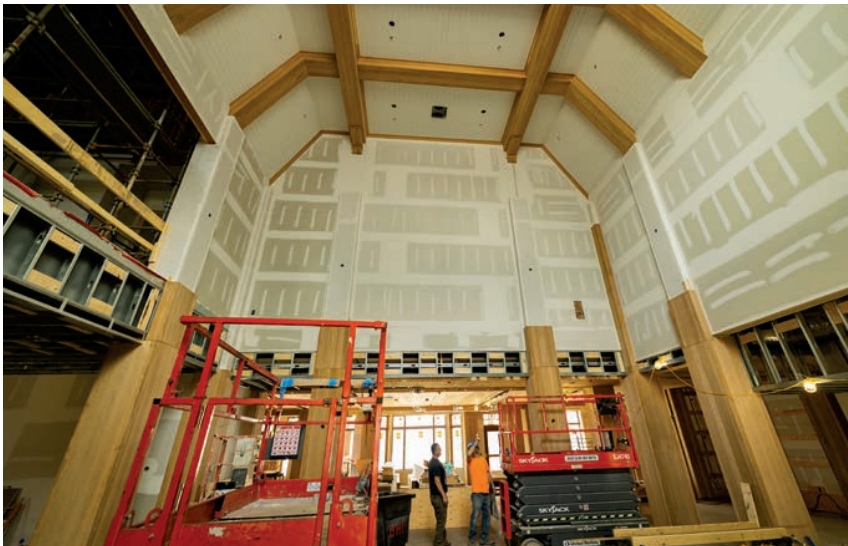
During a tour of The Lake Estate in April, construction was under way on its grand public spaces.
